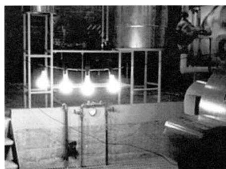
Figure 7.1 Experimental Breeder Reactor-1. By illuminating four light bulbs
